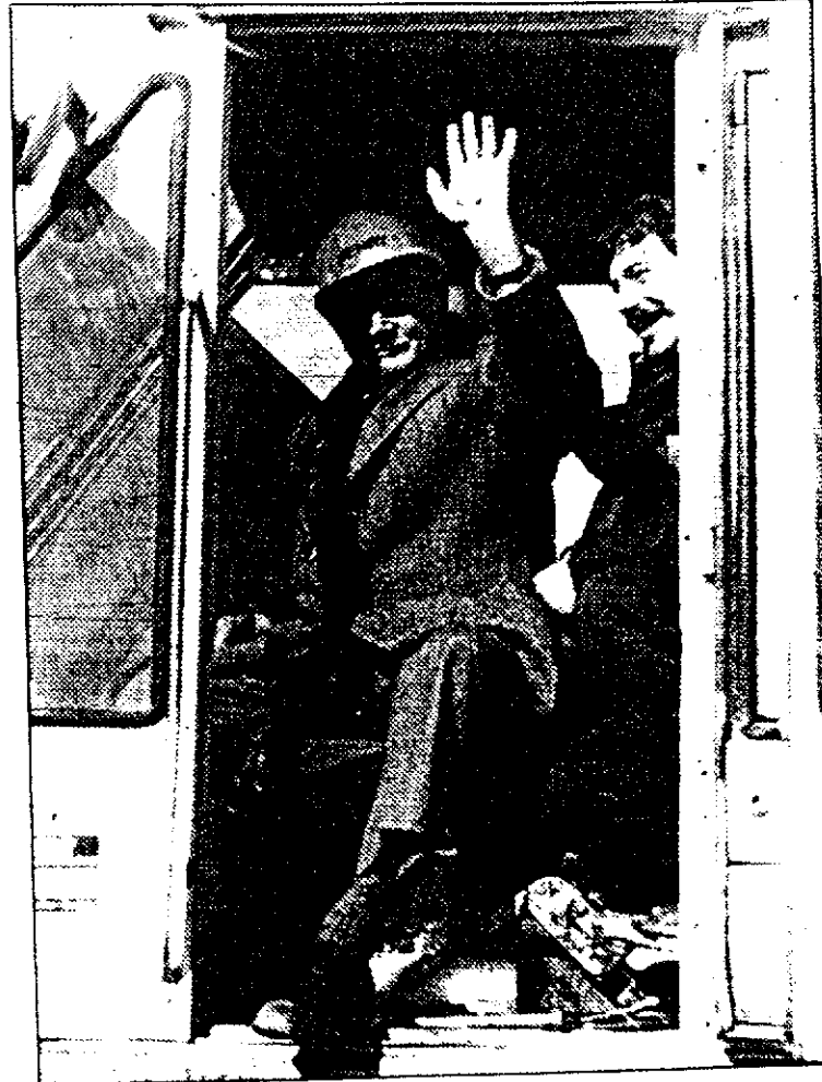
Redekopp on demolition day.
