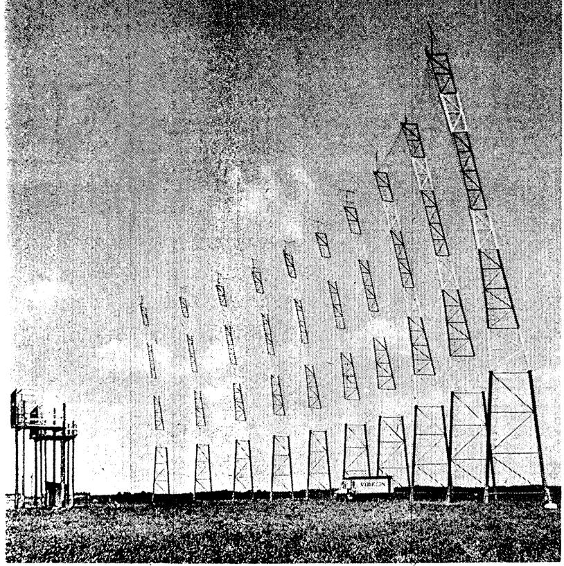
These giant reflectors will enable area residents to receive programs from television stations 184 miles away. The reflectors gather the signals from the air and concentrate them on a focal point. There they are picked up and fed to electronic
