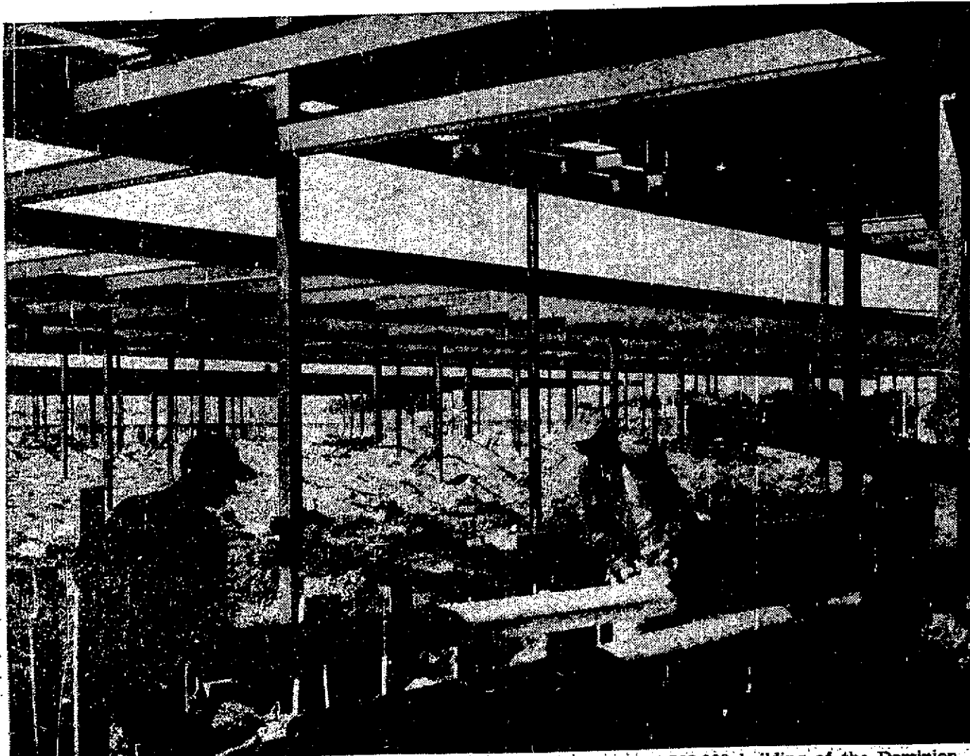
A new addition to East Kildonan's growing industrial area is this $1,500,000 building of the Dominion Envelope and Carton company, now under construction.
