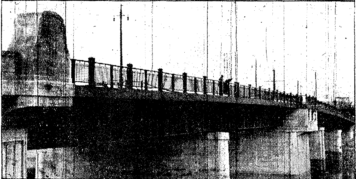
Two views of the new Norwood bridge, which will be formally opened for traffic Saturday afternoon, together with the new bridge over the Assiniboine river, are shown above. The upper photo shows workmen putting the finishing touches on the lighting equipment of the bridge, and the lower shows a striking side view of the structure, snapped by the Free Press cameraman from the banks of the Red river.
